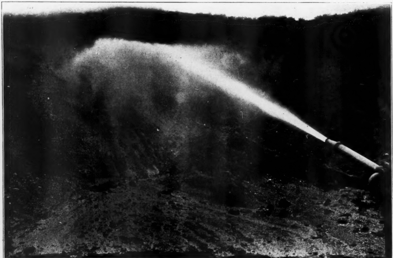
The Bank is Broken Up and Washed Down by the Stream of Water as Shown and Then Picked Up by the Dredge Pump
